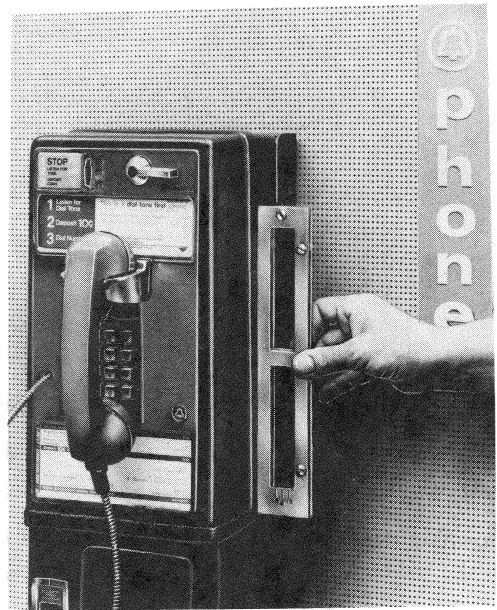
Fig. 10—KS-22473 Leveling Device Being Used to Check Side Alignment
